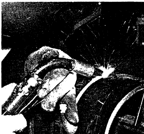
Fig.3-14 Gas metal arc welding
