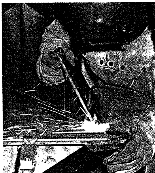
Fig.3-10 Shielded metal arc welding
